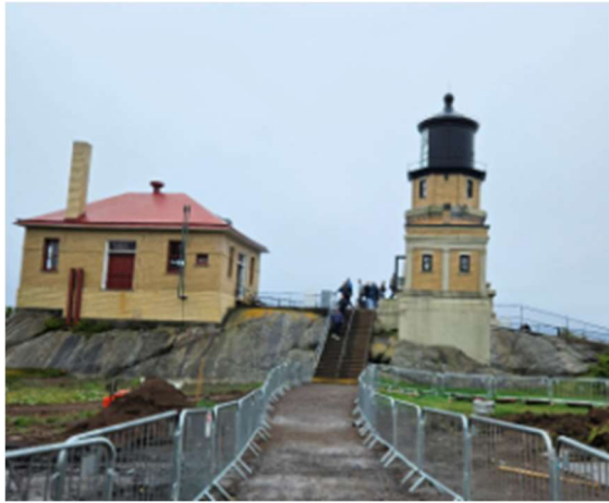
Split Rock Lighthouse
