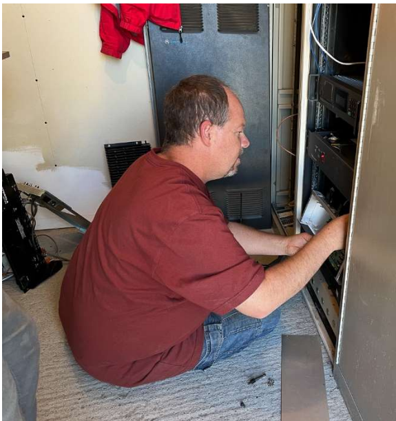
KE7NLU installs the repeater controller.
